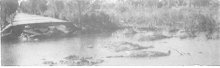
The Buchanan River drains a lot of country north and north east of Wagin. Here the river washed out Great Southern Highway near Piesseville. Taken in the mid fifties.
